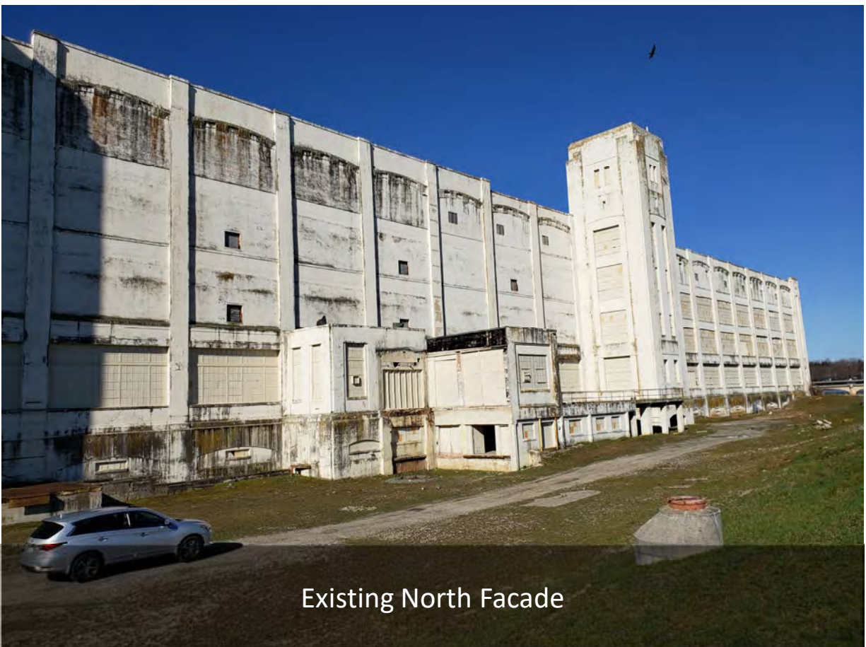
Existing North Facade
