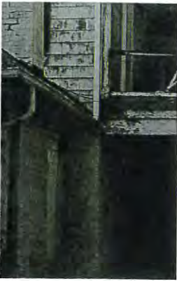
Detail of brick and cedar shakes
