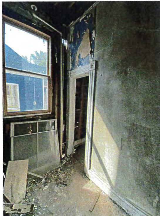
Lower level room on left side of house
