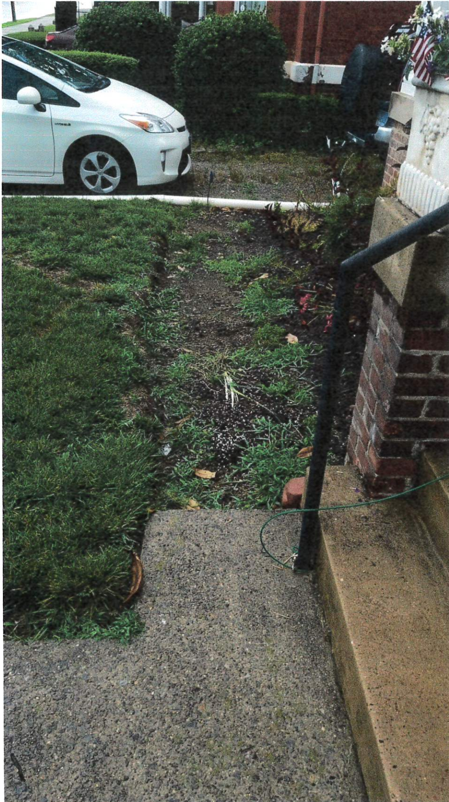
Figure 4 Area for Replacement of Walkway (front left of entry)
