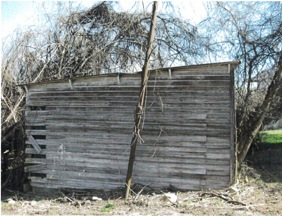
Original shed building, located on my property line, this is looking east. The side to the right was facing the street, but behind the demolished house. I refer to this as the South Elevation later in the document,
