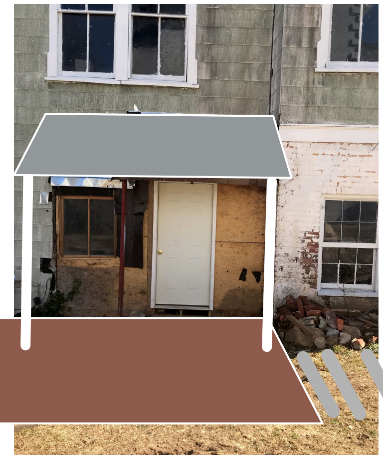
Ugly & useless door overhang, causing more rot and decay on structure
