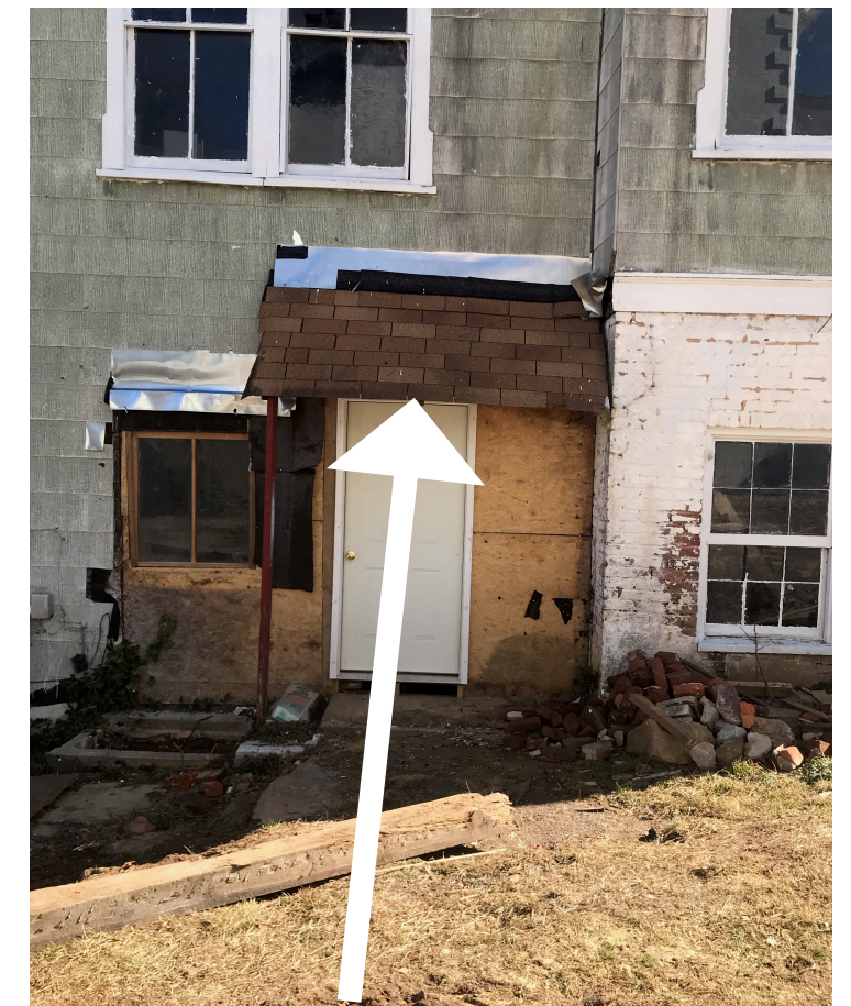
Ugly & useless door overhang, causing more rot and decay on structure
