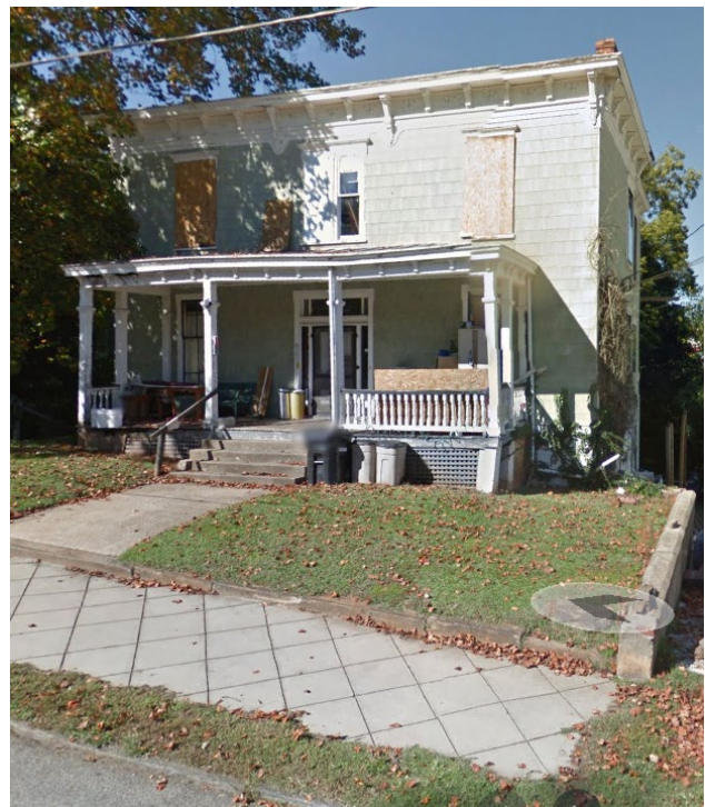
Figure 1 - Street view of 858 Pine Street.
