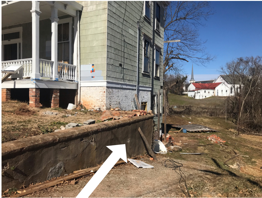
Existing Concrete retaining wall, this side slopes off about 10-12 feet
