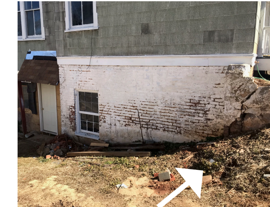
Remnants of concrete/brick retaining wall & steps which were removed.
