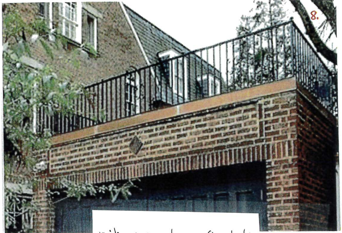
railings around a rooftop deck
