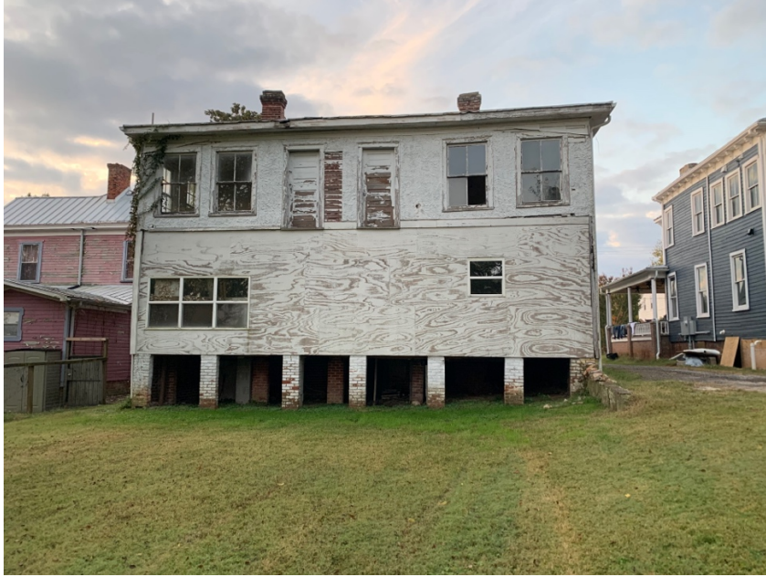
Existing rear façade, windows, & doors
