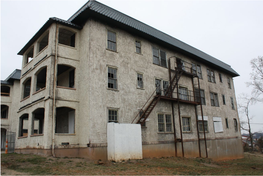
Photo 5: Side (East) Elevation, view NW
