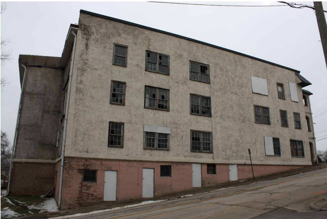
Photo 2 West Side Elevation, view SE
