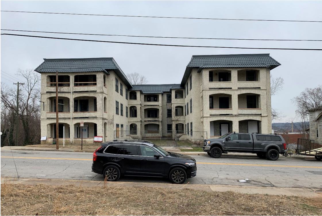
Photo 1: Front (South) Elevation, view north
