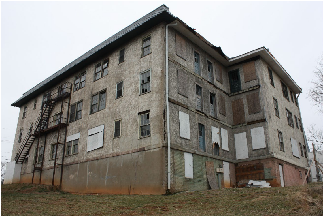
Photo 4: Rear (North) and Side (East) Elevations, view SW
