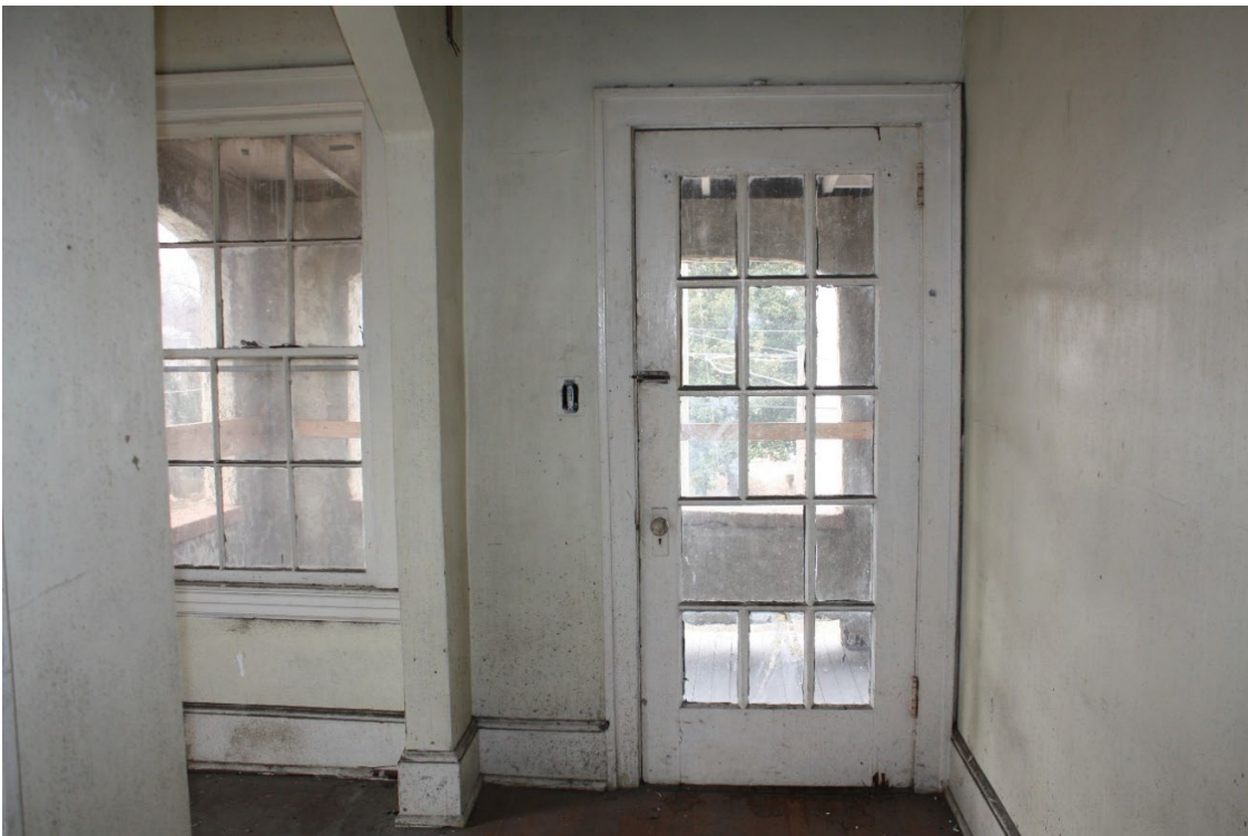
Photo 16: First Floor Plan & Finishes , typical balcony door facing Jefferson Avenue
