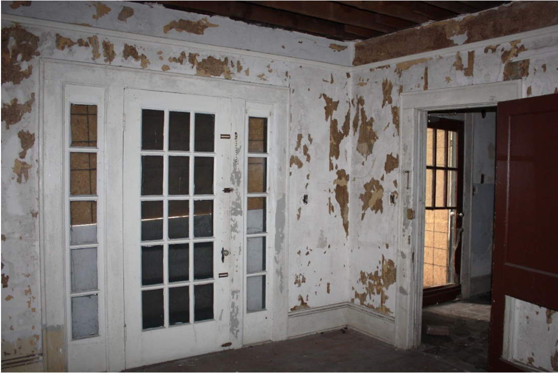
Photo 15: Exterior Doors , typical balcony door facing central courtyard
