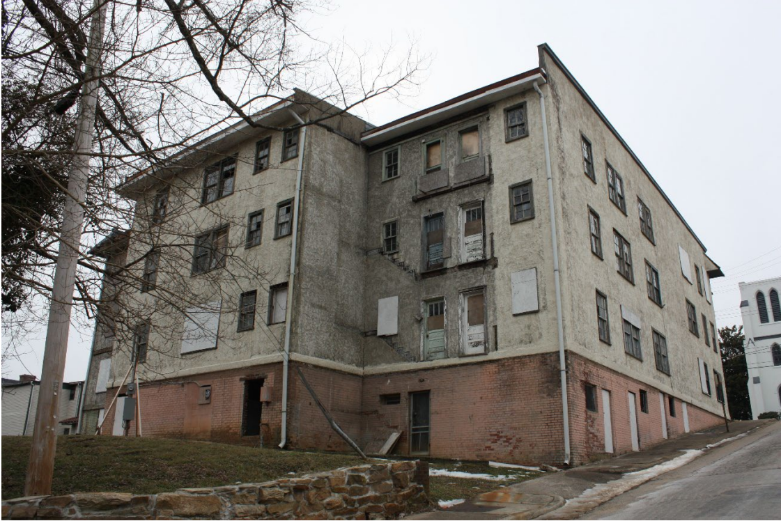
Photo 3: Rear (North) and West Side Elevations, view SE
