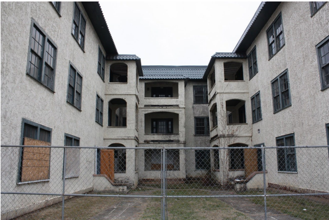
Photo 6: Front (South) Elevation, central courtyard, view north
