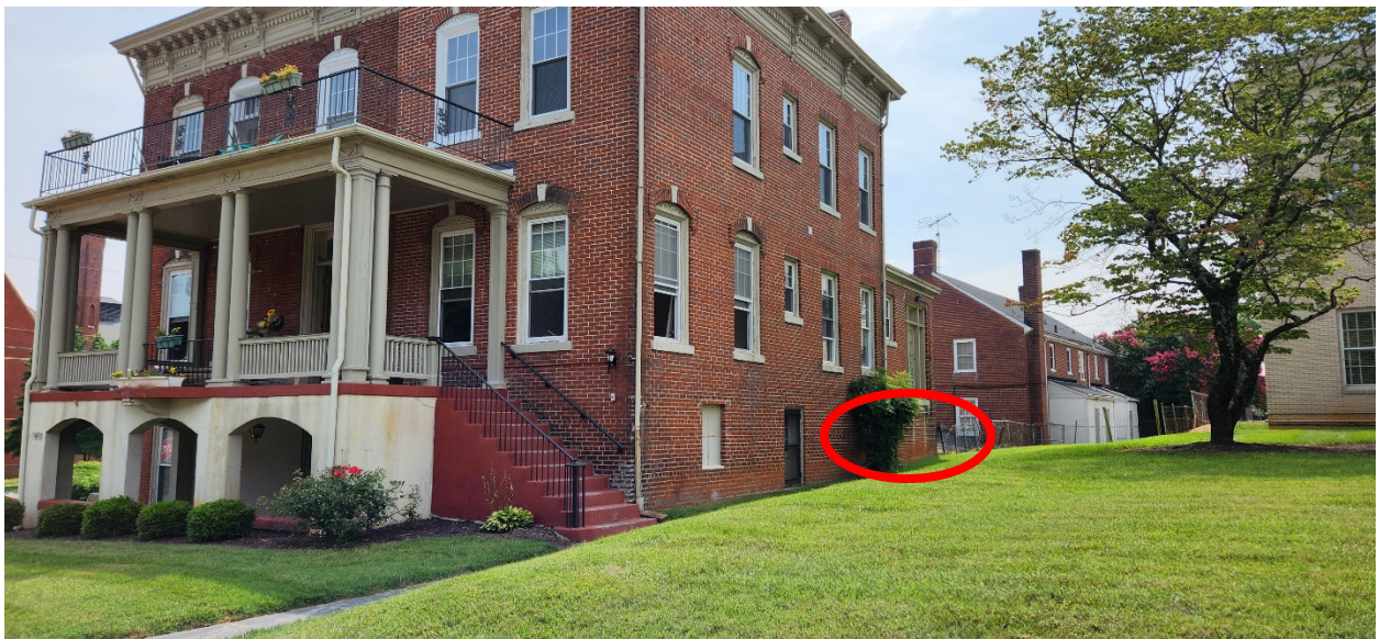
View of area from Main Street sidewalk.
