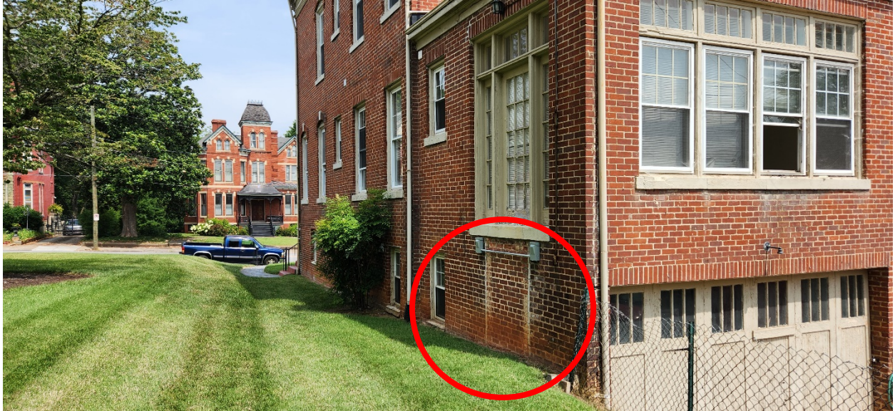
Location of equipment installation
