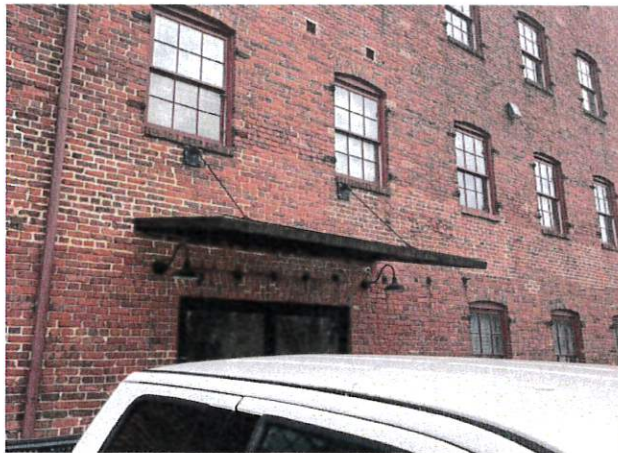
Awning Examples (done by Bailey Spencer Welding)
