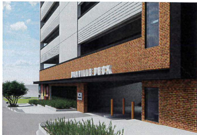
SOUTHWEST CORNER LOOKING FROM N. UNION ST. SCALE: NTS
