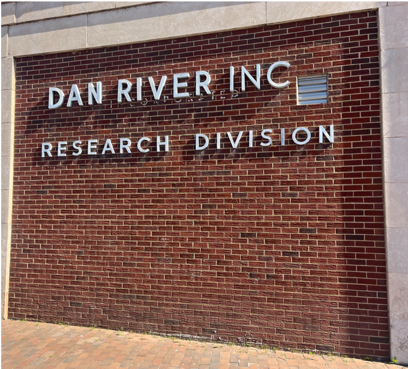
EXISTING SIGNAGE (BRIDGE STREET FACADE)
