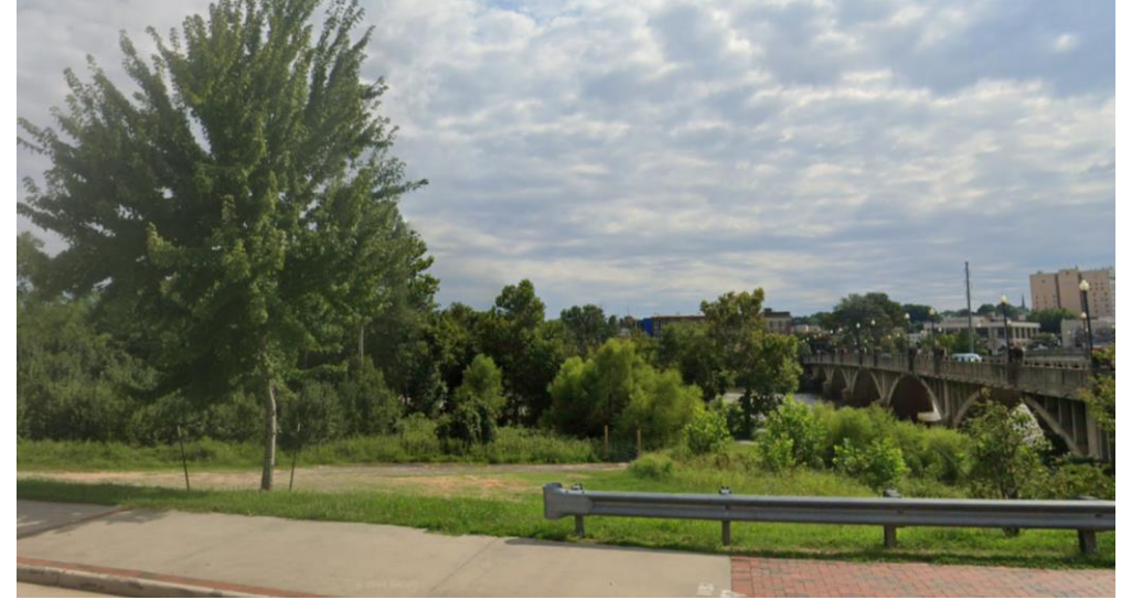
100 River St – looking South
