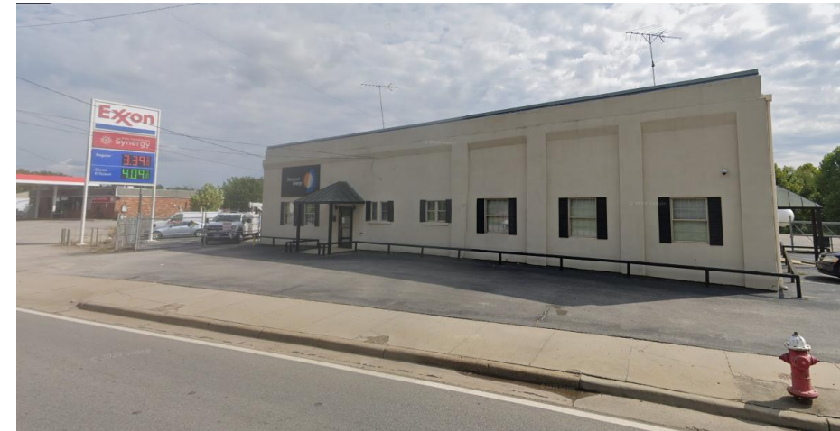
200 River St – looking South
