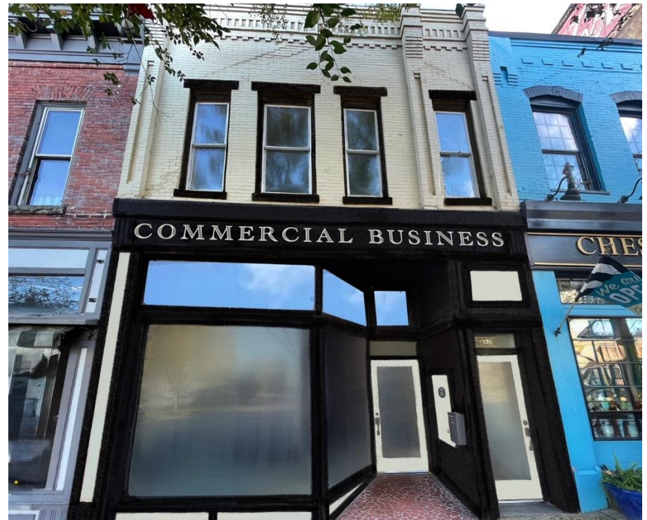
527/527 Main after repair and new paint
