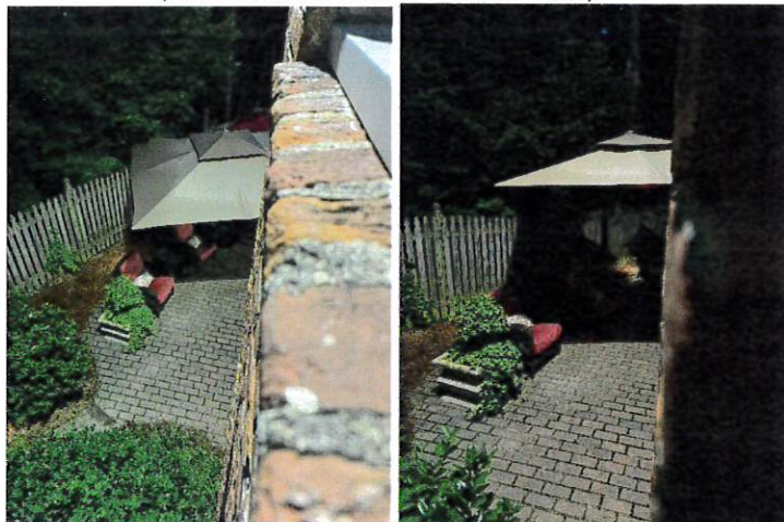
No view of the Porch from 90° angle (Note: second-floor & Ground view)
