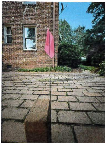
Porch Corner 1' from End of the existing house corner
