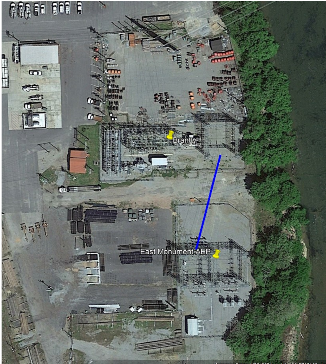
Brantley Substation Delivery Point-1040 Monument Street
