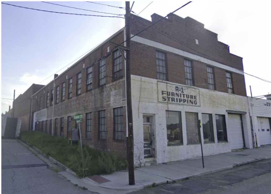
Photo of Subject Property (Pre-Renovation)
