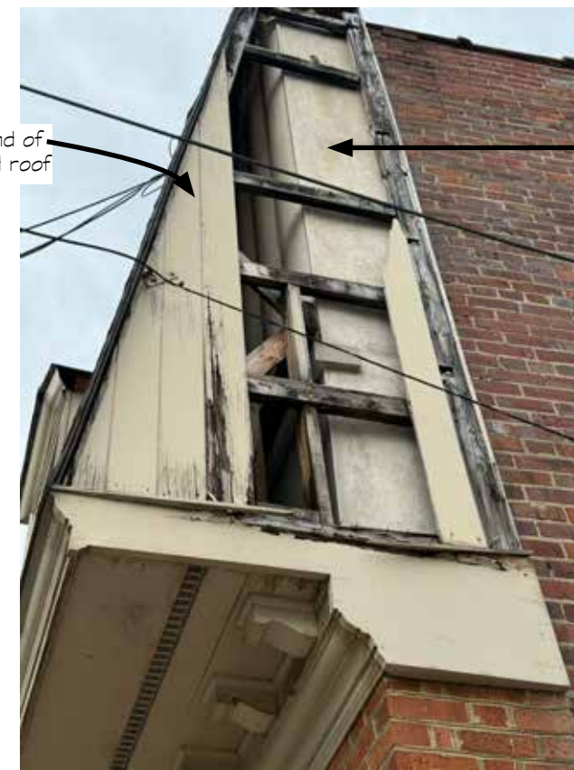
EAST END OF MANSARD ROOF
