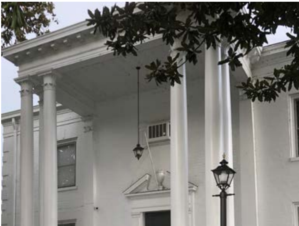
Figure 2.23. Although the placement of a wall air-conditioning unit on the façade is not ideal, the equipment does not obscure any architectural features, has been painted to match the dominant wall color, and is partially obscured by the portico.
