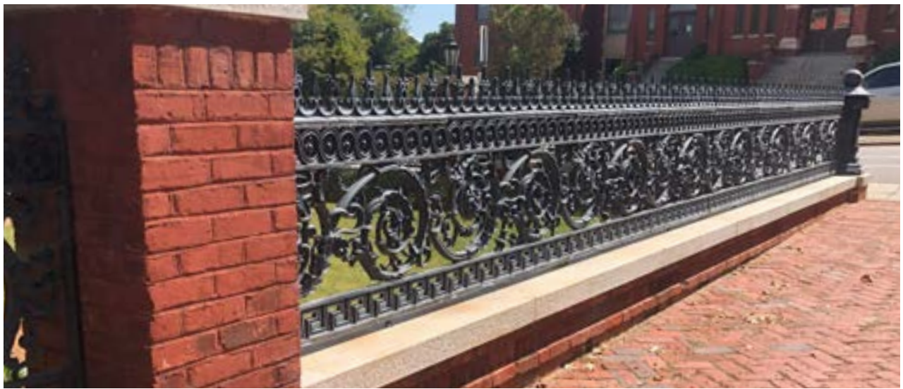
Figure 2.21. This combination fence in the OWE has a masonry base and wrought iron cresting.
