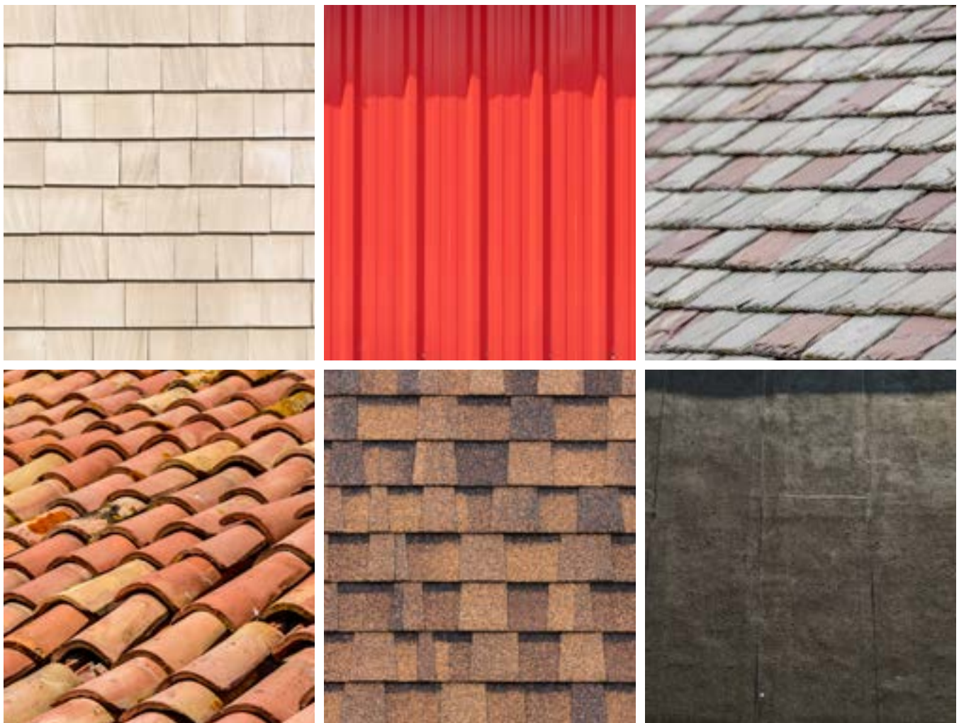
Figure 2.5. Samples of historic roofing materials, from top left to bottom right: wood shingles, standing-seam metal, slate tiles, terra cotta barrel tiles, asphalt shingles, and rubber membrane for flat roofs.
