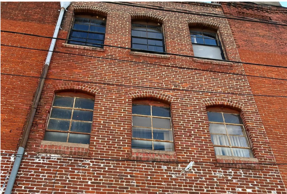
Photo 4H: Windows, Sections C & D, non-historic steel windows (note presence of altered sills)
