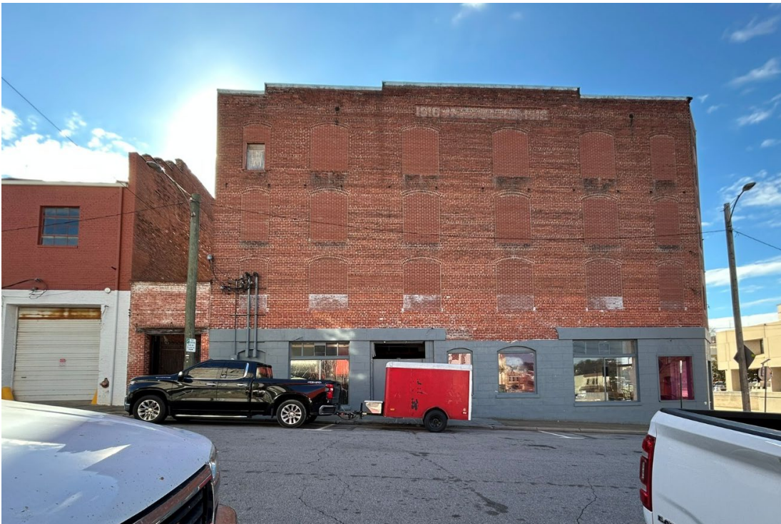
Photo 2: East Elevation, view West from Lynn Street
