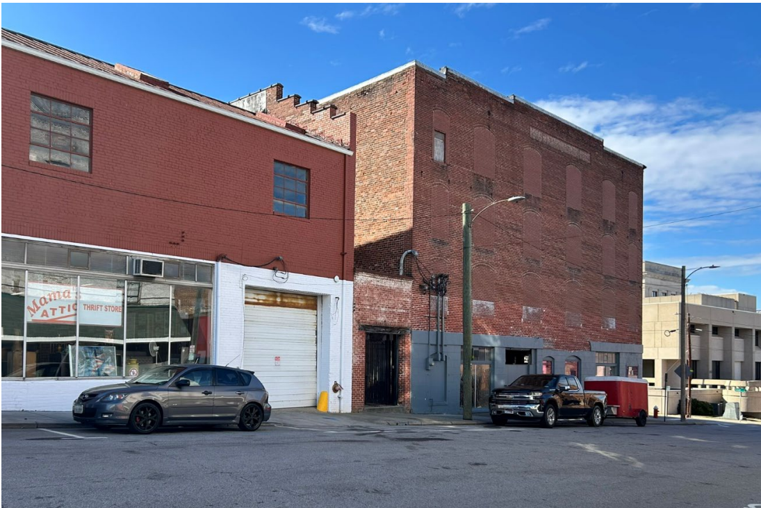
Photo 6: East and South Elevations, view Northwest from Lynn Street
