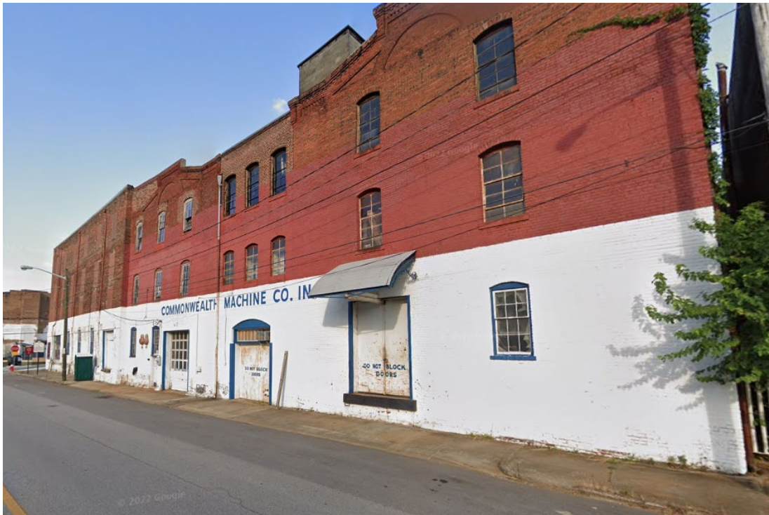
Photo 4A: Exterior Brick Walls, North and West Elevations, Google Streetview 2019 showing painted walls
