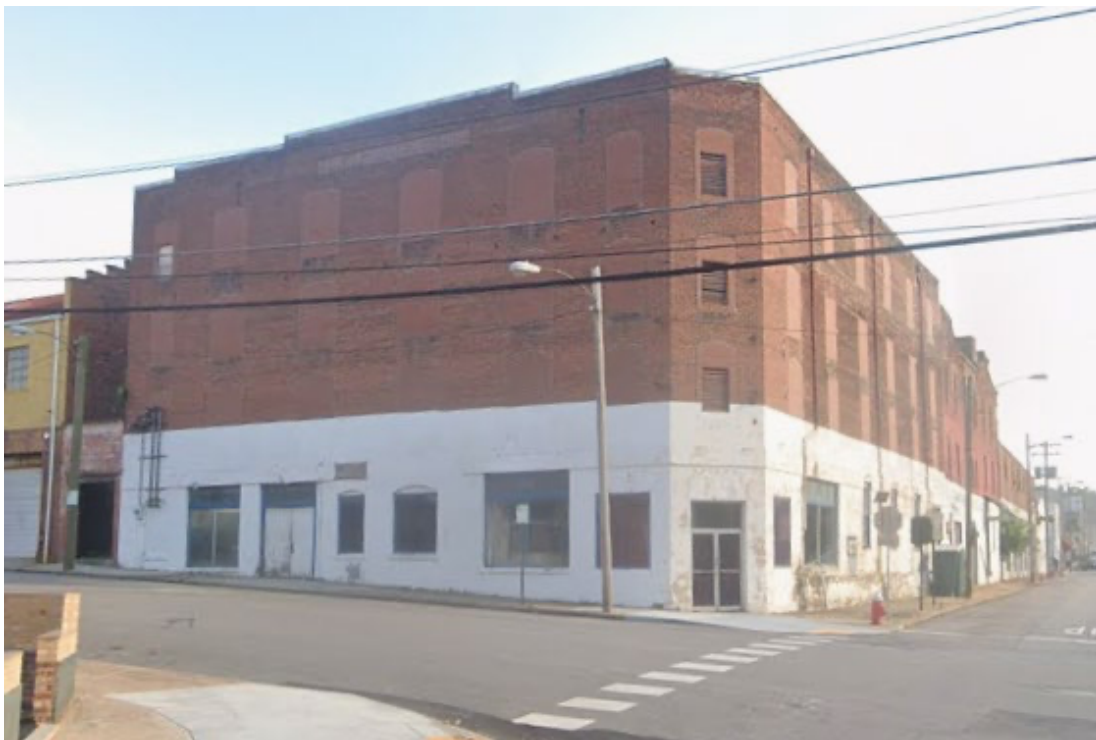
Photo 4B: Exterior Brick Walls, North and East Elevations, Google Streetview 2019 showing painted walls
