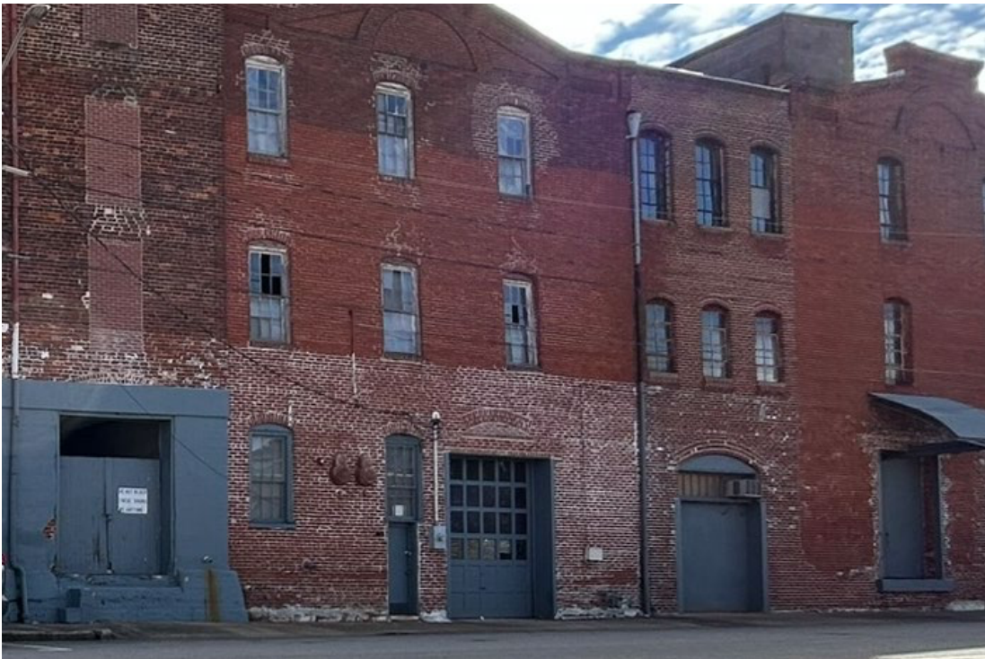
Photo 4J: Exterior Doors, Sections A-D, masonry arches denote extents of historic freight openings
