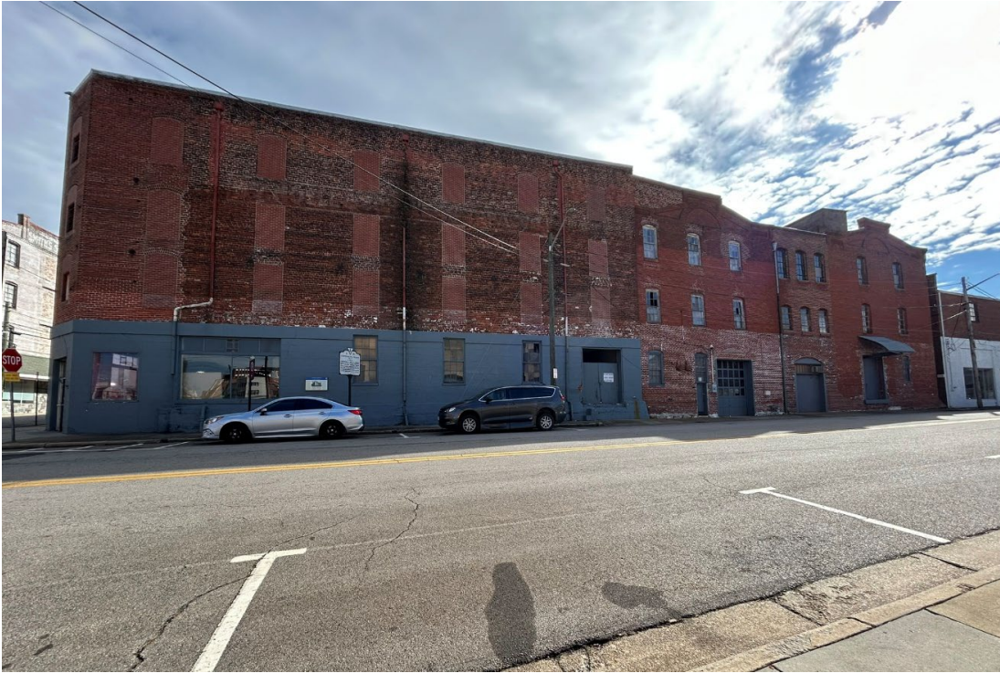
Photo 3: North Elevation, view South from Loyal Street
