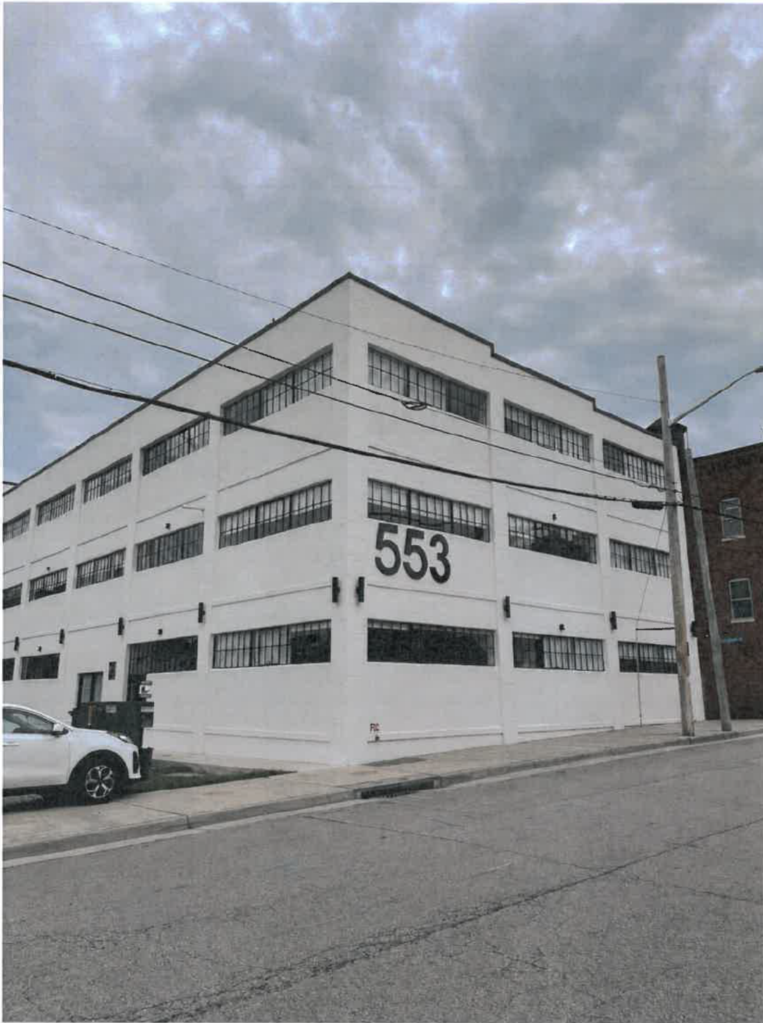
**Picture taken 8/27/26. Altered to show building with a single sign facing Lynn St.
