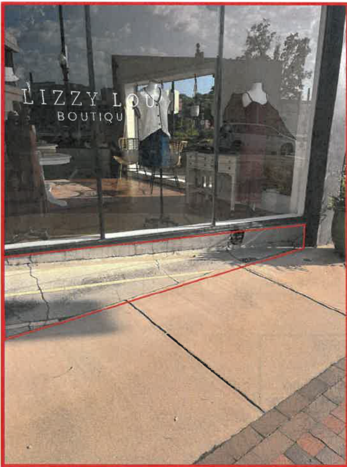
Current condition of terrazzo
