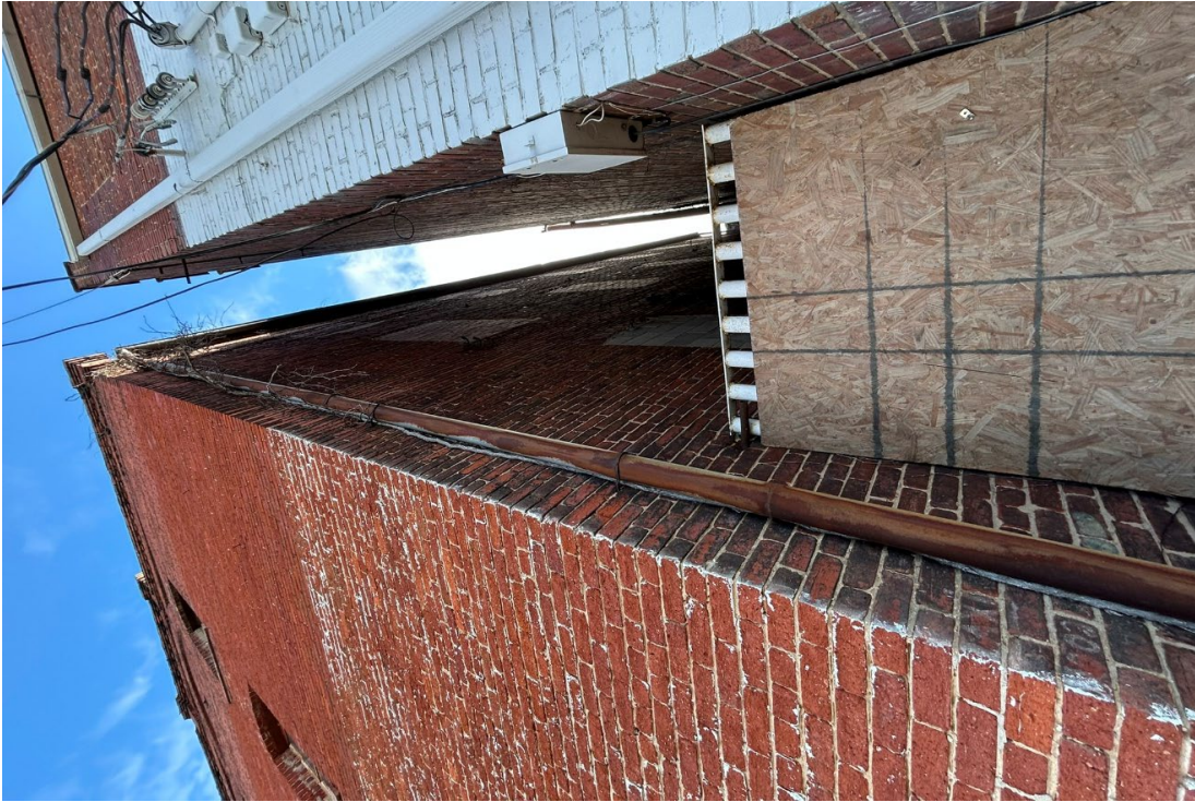
Photo 5: West Elevation, view South into Western Alley, from Loyal Street
